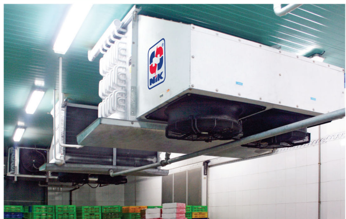
Spiral freezer ammonia unit coolers AND-S Capacity range 28.6 to 365.9 kW Fan diameter 630 or 710 mm NO. of fans 2,3,4 or 5 fans Fin spacing 6,8,10,12,15 or 12/15
