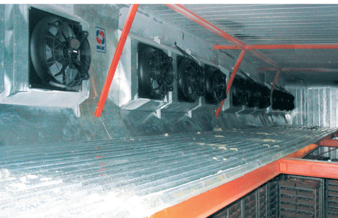
Tunnel freezer ammonia unit coolers AND-T Capacity range 48 to 295 kW Fan diameter 630 or 710 mm NO. of fans 2,3,4 or 5 fans Fin spacing 6,8,10,12,15 or 12/15
