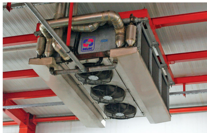
Angle type ammonia unit coolers AND-A Capacity range 48 to 203.3 kW Fan Diameters 630 or 710 mm NO. of fans 2,3,4, or 5 fans Fin spacing 6,8,10,12,15 or 12/15
